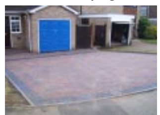
The finished driveway completed and sealed
